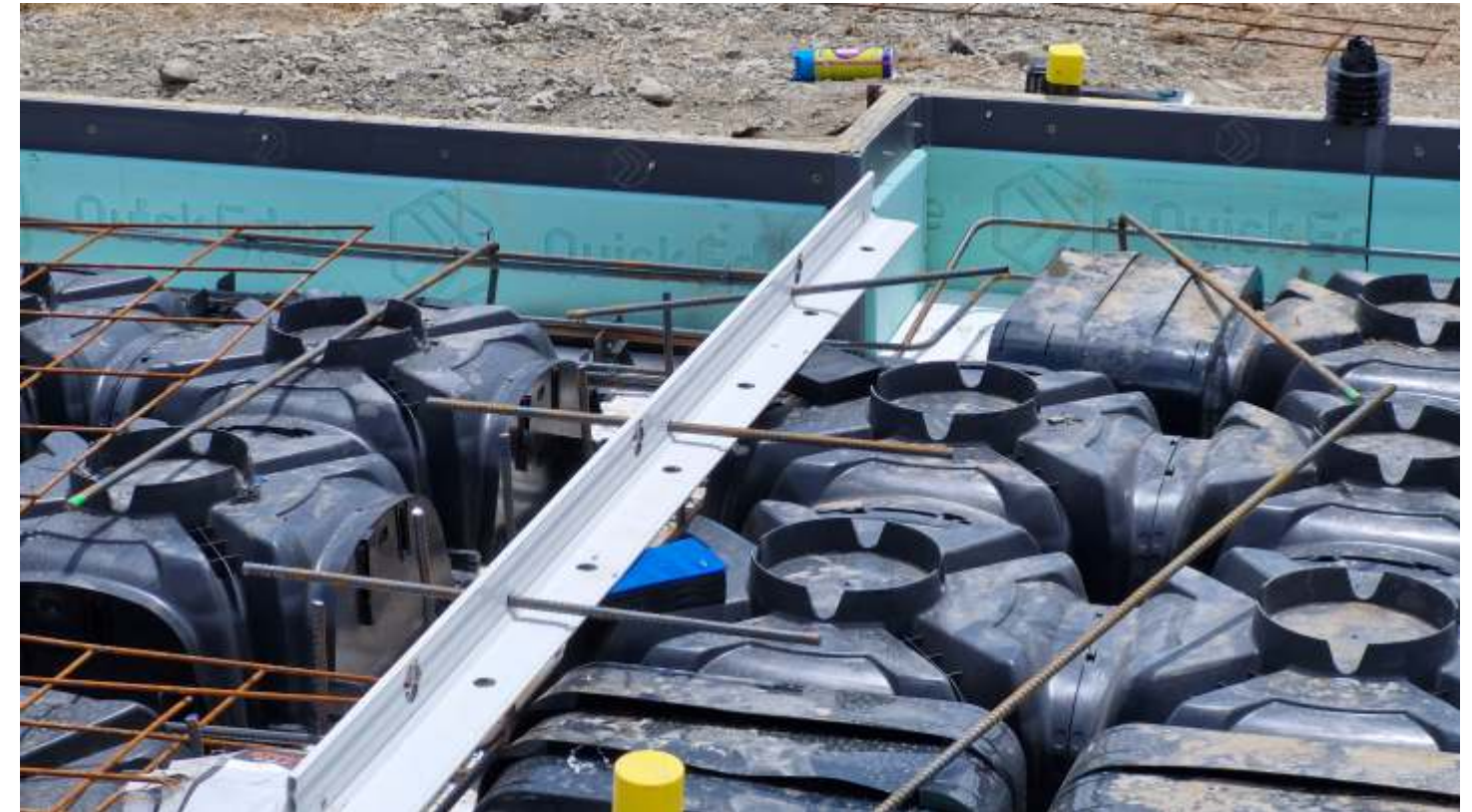
Image provided shows free joint under construction.
